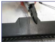
Cut holes to allow cable access
